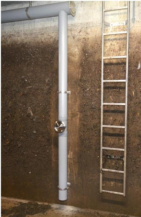
*Figure 2: Extraction pipe*
