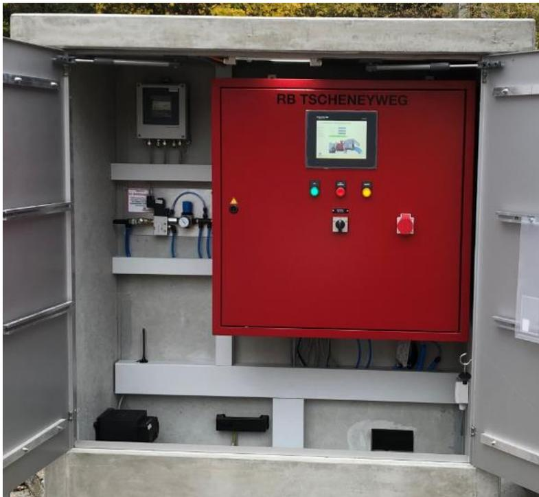
Figure 7: ALLinONE rainwater basin control with pneumatic discharge control in the control cabinet Biel BE/CH LxWxH 800x800x250mm.
