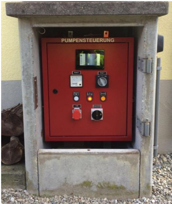
*Figure 6: ALLinONE for 1 wastewater pump using the example pumping station in Meiringen BE/CH; Cabinet WxHxD 500x600x250mm retrofitted in an existing concrete cabin.*
