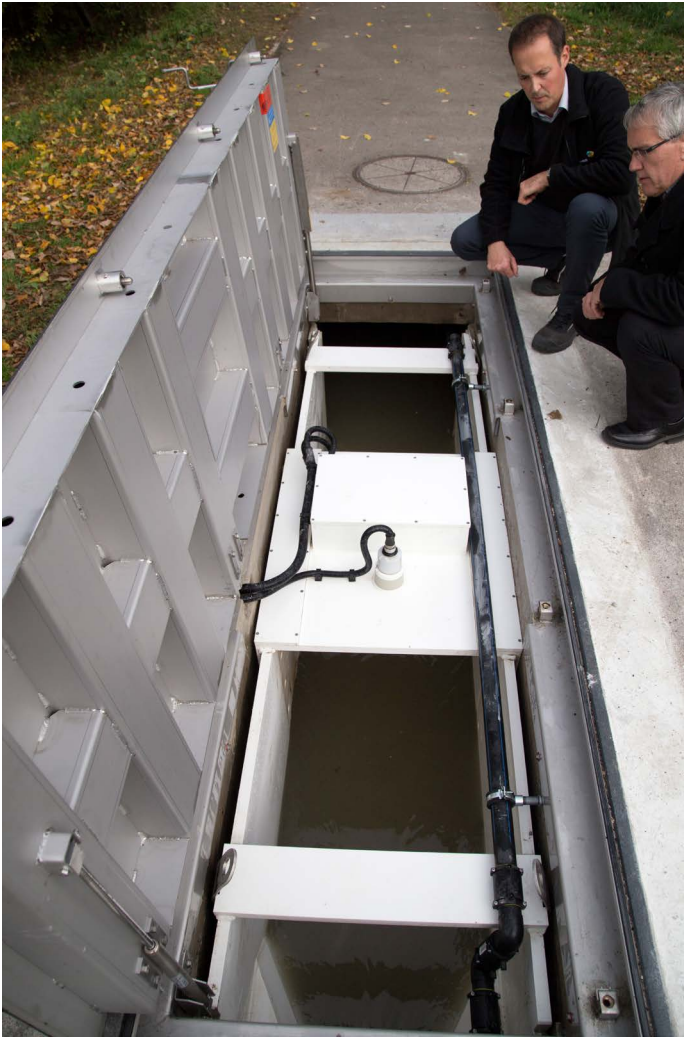
Thomas Di Lorenzo and Andreas Zingg (STEBATEC) are seen watching the newly fitted part-filled permanently installed flow measuring point at a trunk sewer.
