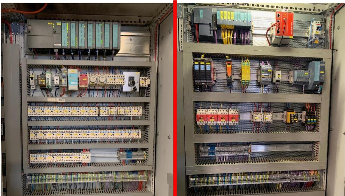
Figure 1: Left before the retrofit / Right after the retrofit
