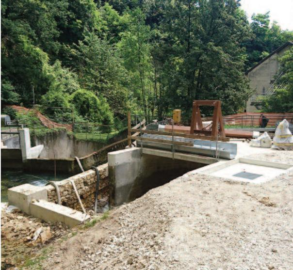
Situation before the installation of the new screen. The hoses in the picture evacuate water.
