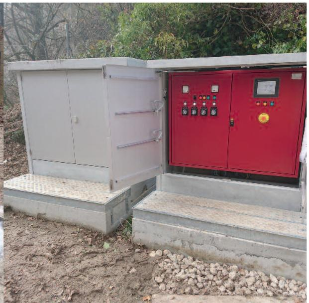
Hydraulic unit and control cabinet are securely installed in concrete booths.
