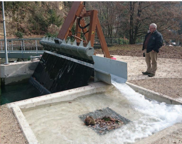
The floating trash, which the cleaning machine lifts into the flushing conduit, is flushed into the concrete basin with bottom screen.
