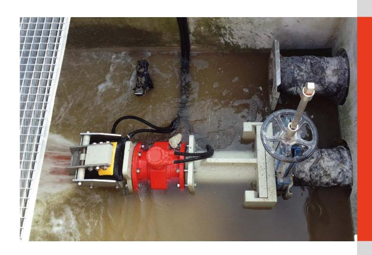
The Oberregenbach sewage treatment plant of the town of Langenburg (D) is located between Stuttgart and Nürnburg and treats the waste water of about 1,800 inhabitants. Located on the foot of a slope, the water from the storm-water basin runs down a steep canal. Before the STE-BATEC drain controller was installed, the waste water was slowed down by a mechanical scale throttle before it entered the sewage treatment plant.
