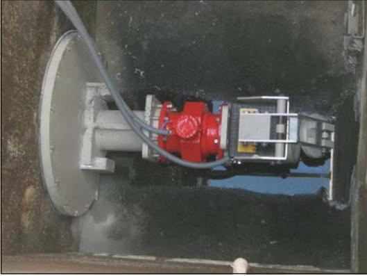
*Pneumatic outflow controls of different designs*
