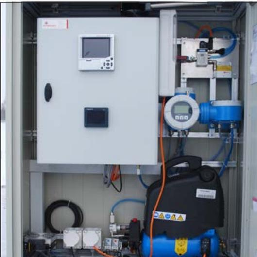
*Free-field aluminum cabinet for pneumatic outflow control.*
