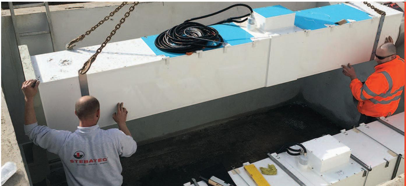
One of the two calibrated measurement channels are being installed for inflow measurement in the shaft constructed for that purpose. The other one (bottom right) is already in place.
