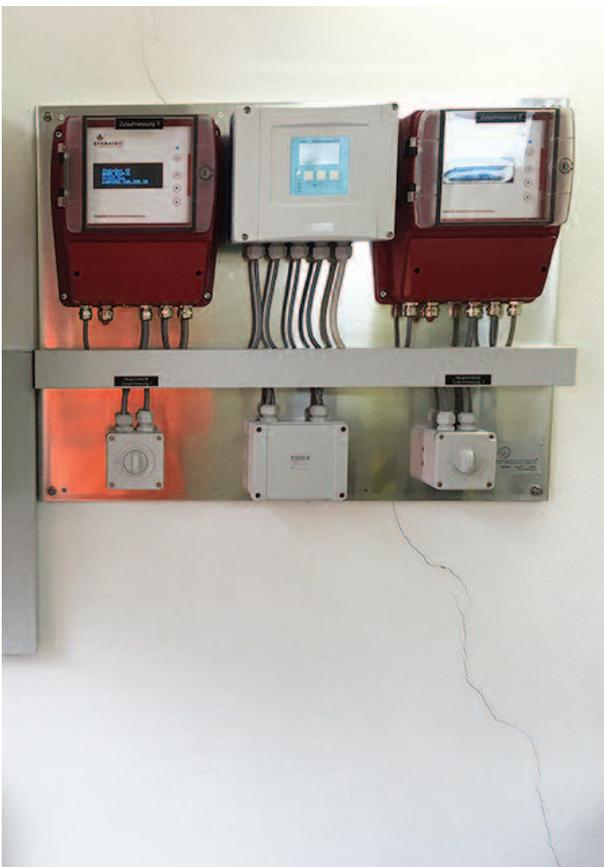
The measurement transducers transfer data to the SCADA system and optionally via GPRS to an external maintenance contractor.
