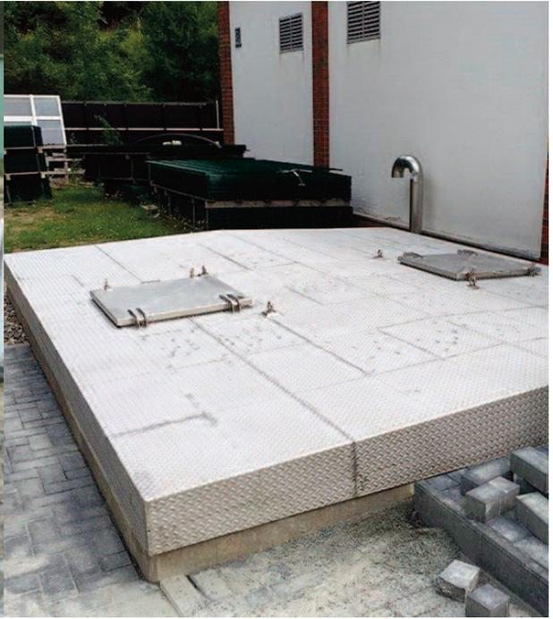
The finished shaft with the cover and the access openings for maintenance and inspection.
